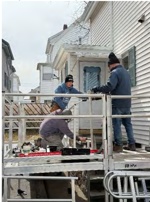
Diamantina's Ramp Install – New Bedford
