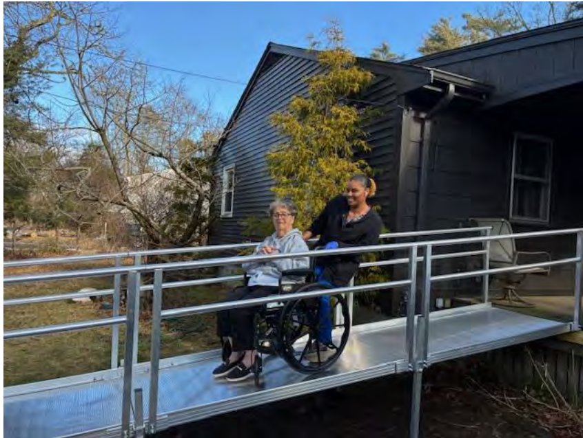
Nancy's Ramp Install – New Bedford
